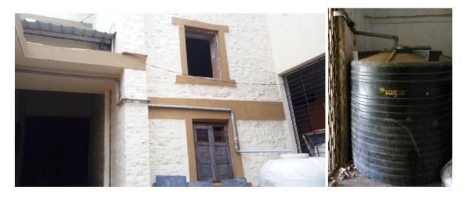
Photo 6-RWH system provided with centralized storage tanks.
