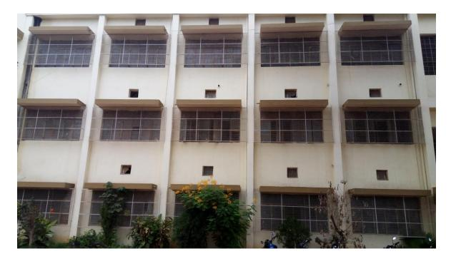
Photo 5-Large windows provided for natural ventilation reducing power consumption.
